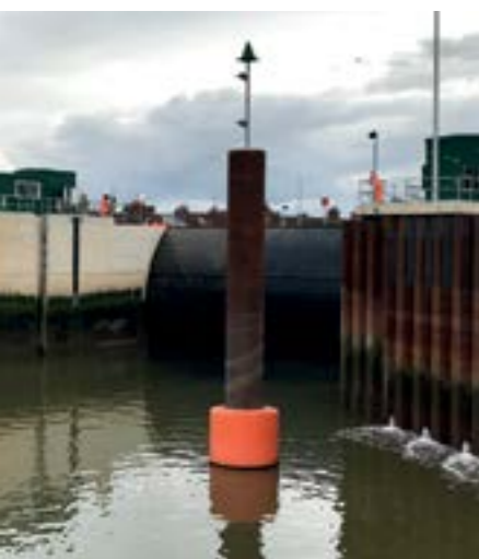
Below: Boston Barrier is a single rising sector gate that protects the town of Boston, Lincolnshire (UK). The barrier became operational in 2020 with the remaining parts of the project due to complete in 2022
