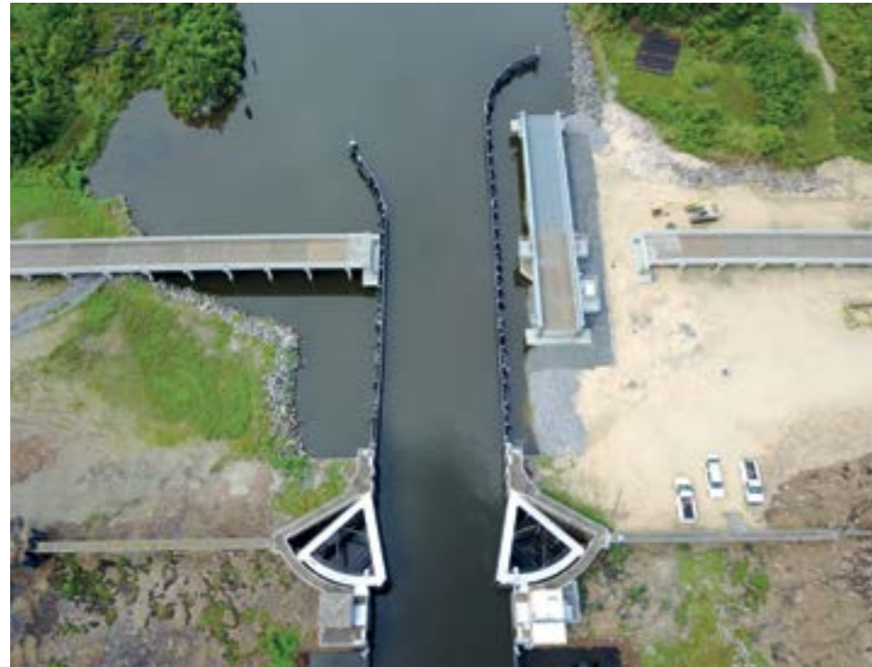
Right: The Bayou Bienvenue Sector Gate is part of the Hurricane and Storm Damage Risk Reduction System that protects New Orleans. The system was built by the US Army Corps following Hurricane Katrina in 2005. It is maintained and operated by the South Louisiana Flood Protection Authority East
