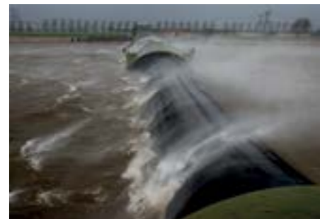
Below: Ramspol Barrier - The Ramspol, operational since 2002, is located in the north-east of the Netherlands. It is an inflatable dam to protect against high water from the IJssel lake
